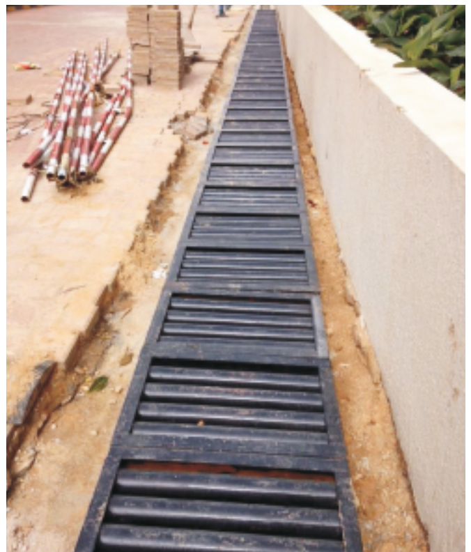
MS Drain Cover fabricated by Everest after laying
