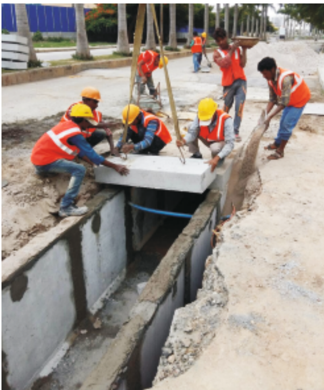
Cover Slab suitable for Fire Tender load being laid over hydrant
