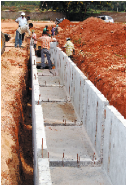
Trench sections being aligned before joining
