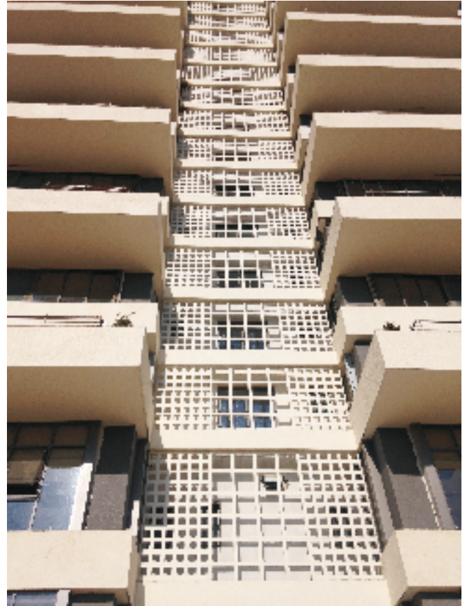
Screen after fixing over service area
