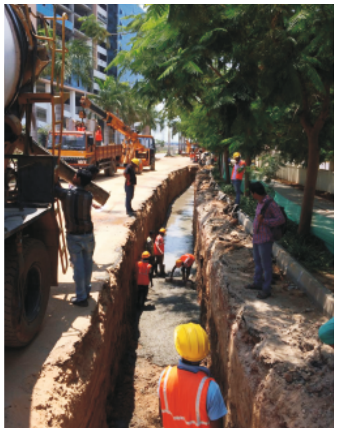
Concrete levelling in progress
