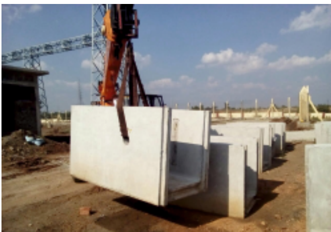
Drain Lifting by crane
