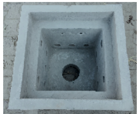
Perforation for cable joint
