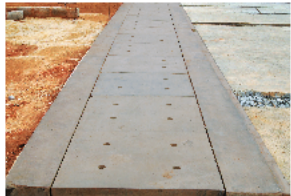
Cover Slabs laid in position
