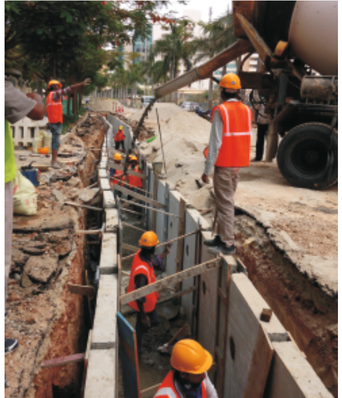
Joining of drains in progress
